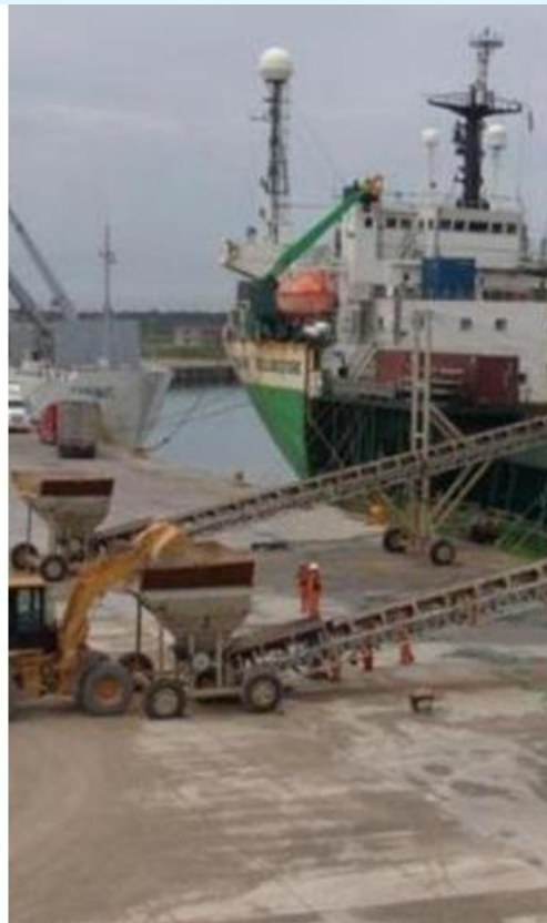
Stone Handling to Subsea Construction Projects.
